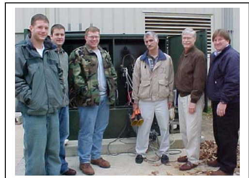
Standing a safe distance from REMC's transformer behind the YMCA are (left to right) Kevin Snyder from Ottawa, OH; Doug McNeill from Trafalgar, IN; David Pruss from Farmer's Retreat, IN; Craig Burgi, marketing director with Steuben County REMC; Dr. Larry Samuelson, TSU professor of electrical and computer engineering; and Jerry Wisdom, project engineer with NiSource Energy Technologies (NET). Not pictured is electrical engineering senior Josh Warner of Oregon, OH. Warner will be working with Samuelson to collect and analyze the data from the power monitor.
